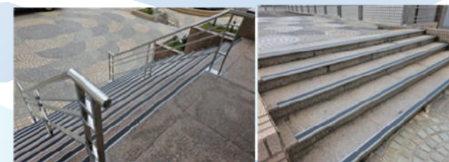
Outdoor ladder handrails and anti-slip safety facilities at Chung-Shing Plant
